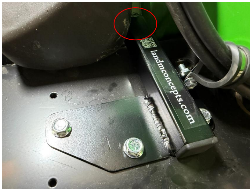
Figure 6 - Mast and cable clamp installed
